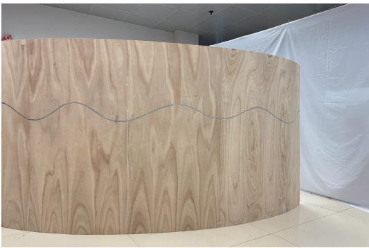
图 20 曲面板曲线型结合缝整体涂胶效果 Fig. 20 Overall glue dispensing effect on a curved plate with a curved groove seam
