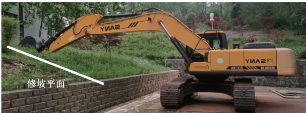
图 10 挖掘机器人最常用的修坡工况轨迹跟踪实验示意图 Fig. 10 Schematic diagram of the trajectory tracking experiment for slope repair condition of the robotic excavators
